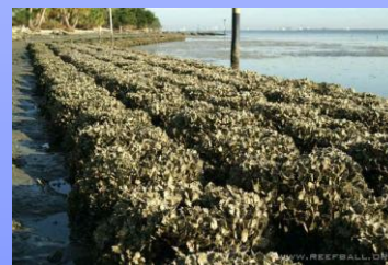
Estuary breakwaters to reduce erosion from boat wash and provide structure for oysters. Photo: Reef Ball Foundation
