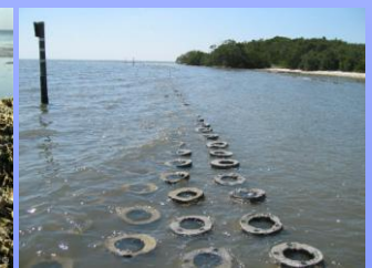
Estuary breakwaters to reduce erosion from boat wash and provide structure for oysters. Photo: Reef Ball Foundation
