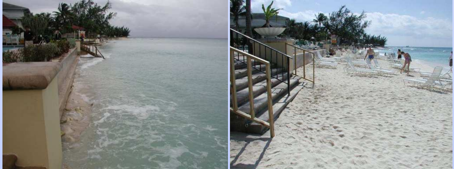
Grand Cayman Marriott Resort, Cayman Islands. Before and after construction of the Reef Ball Breakwater, Oct 2003 and Feb 2003. Photo: Lee Harris
