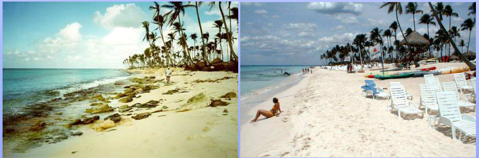
Gran Dominicus Resort, Dominican Republic. Before and after construction of Reef Ball Breakwater, 1998 and 2001. Sand accreted at a rate of 26-44 m 3 /m from 1998-2001. Photo: Lee Harris
